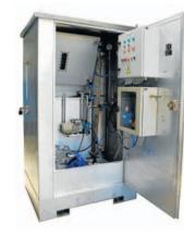
operate within fluctuating levels of groundwater and LNAPL, which means it removes thin layers of hydrocarbon products. In other words, mostly contaminated product is pumped to the surface, which reduces the need for further time-consuming and costly separation of LNAPL and water
